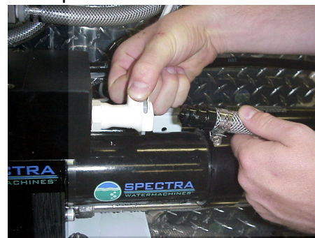
Connecting brine discharge service-hose
