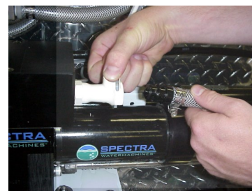
Connecting brine discharge service hose
