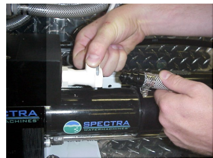
Connecting brine discharge service hose
