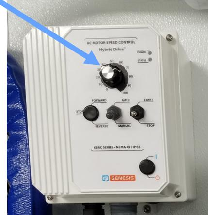
The boost pressure is adjusted with the large knob on the boost pump speed control. You will notice that as you change the boost pressure the sound of the Pearson Pump will change.
