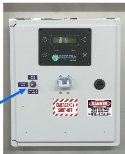
Manual Run Toggle Switch
